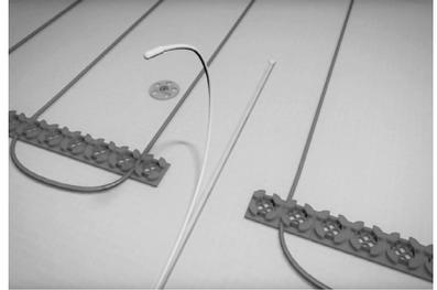
**NOTE:** Do **NOT** run the cold lead wires and the floor sensor in the same conduit.
