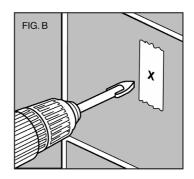
Apply masking tape to the tiles in the area you wish to mark the holes and mark the hole positions through onto the tape (Fig A). Leave tape on tiles to guide drill and using a 6mm masonry drill, drill holes (Fig B) to a depth of ½" before inserting wall plugs.
