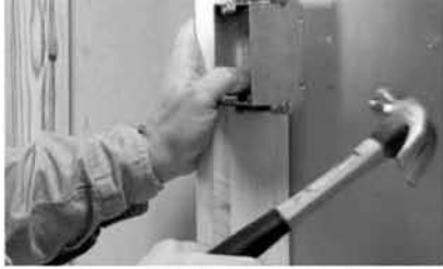
Figure N2. ECB installation
