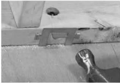
Figure N5. Guards installation
