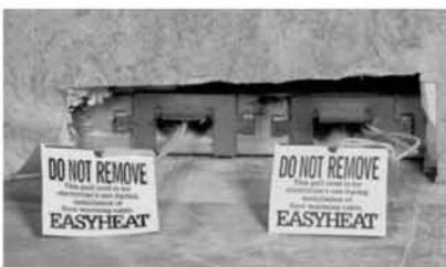
Figure R6. Fish cord installation
