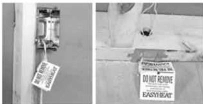
Figure N7. "Do Not Remove" tags installation
